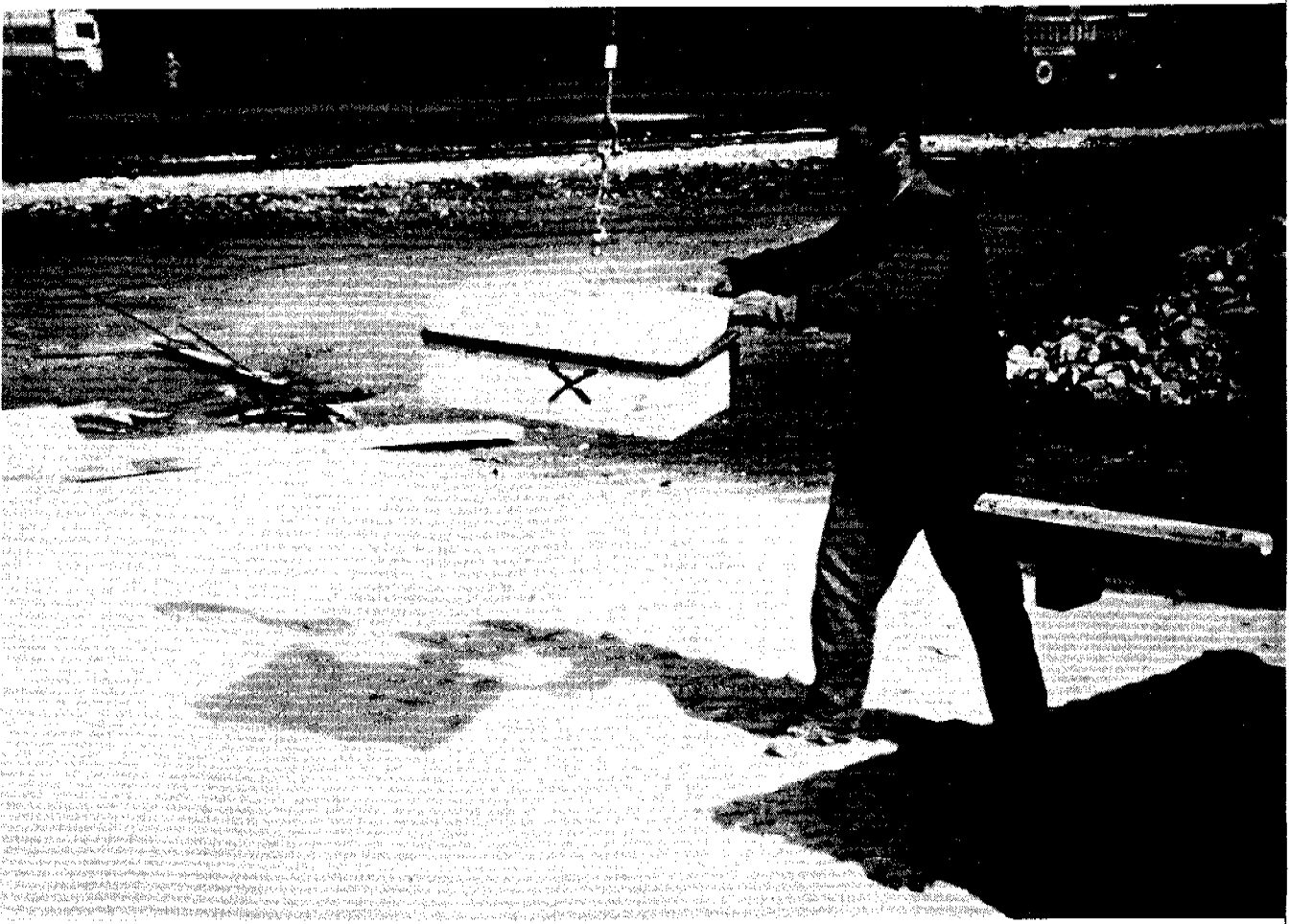
Figure 13 Rubber joints for semi-rigid floating pavement
