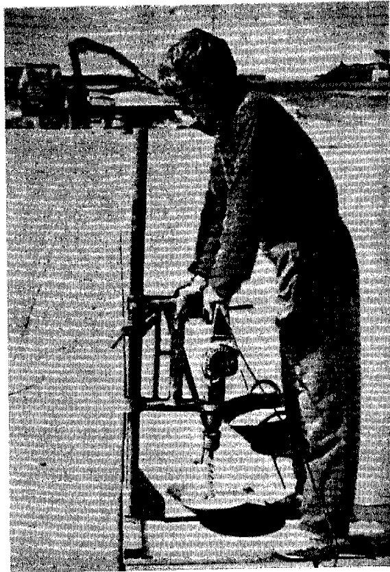
Figure 16 Vibrating roller to settle semi-rigid floating pavement
