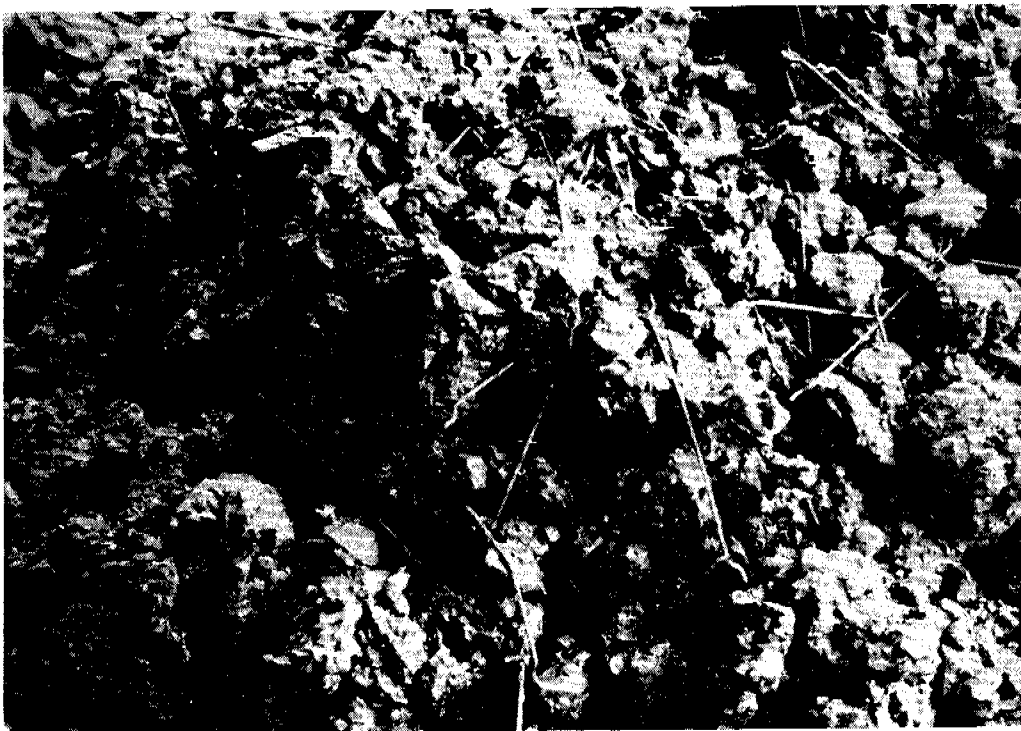
Figure 6 Concrete mix showing dispersion of steel fibres
