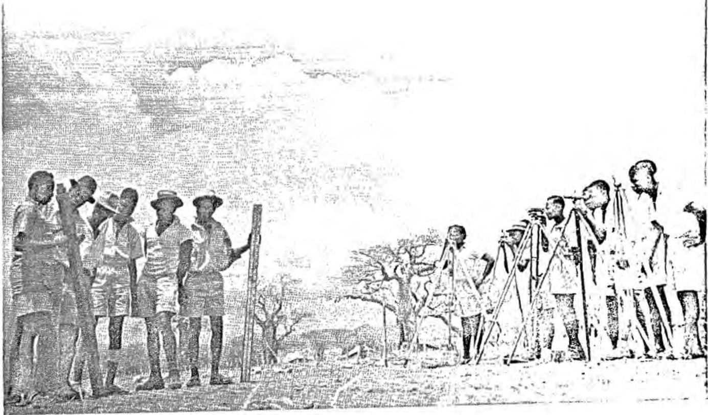
GROUNDNUT SCHEME: TRAINING CLASS FOR AFRICAN SURVEYORS
