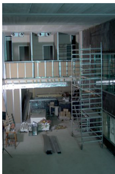
Construction of the courtroom and media centre in 2003 © ICC-CPI
