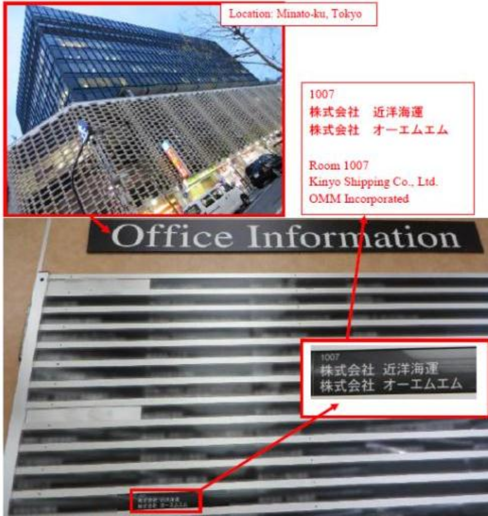
Source: Photos of 28 February 2014 obtained by the Panel
