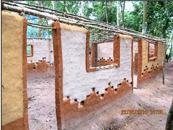
Building identified as a mosque by FARDC, at Madina camp. Photographed by the Group on 22 April.
