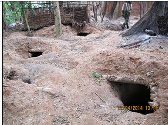
Entrance to bunkers that appear to have been constructed as air raid bunkers, at Madina camp. The Group identified such bunkers at Madina camp but did not see evidence of them at Kabila or AKBG camps. The bunkers appear to have been recently constructed. The Group also identified other underground bunkers that appear to have been used for storage, or as holding cells for prisoners. The Group took this photo on 22 April.
