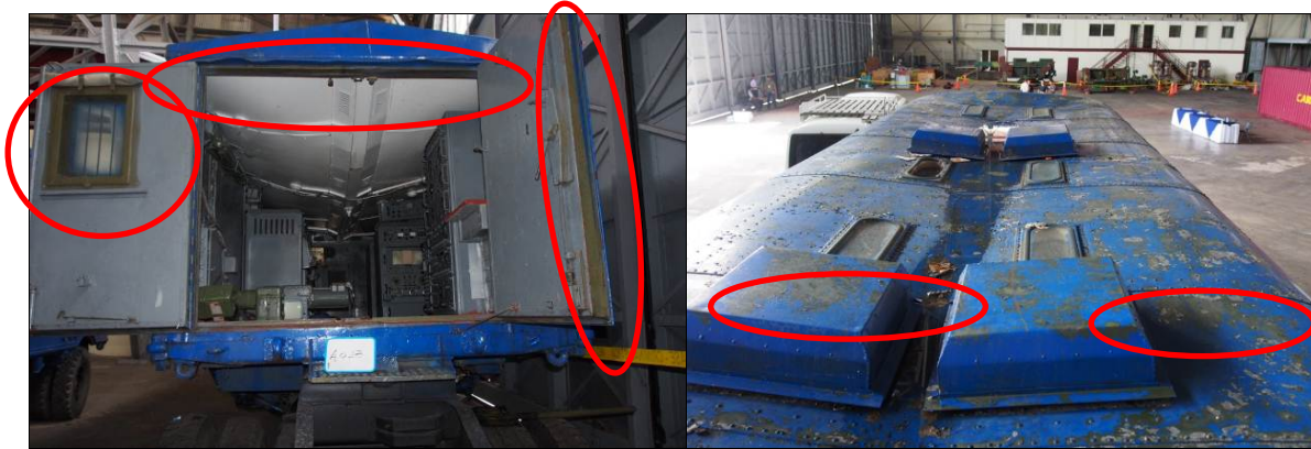
Figure 2: Original paint scheme inside (left) and revealed by damage (right)
