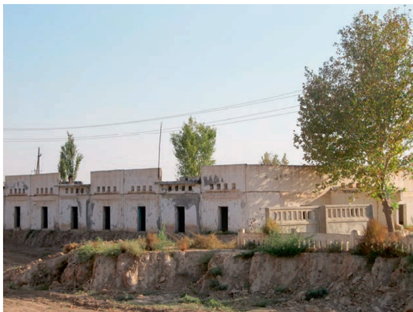
Photo 10.1: Infrastructure damage to tuberculosis ward from mudslide, District Hospital
