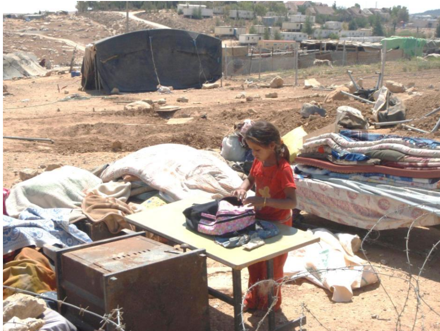
Demolished house in Hebron/OCHA 2011
