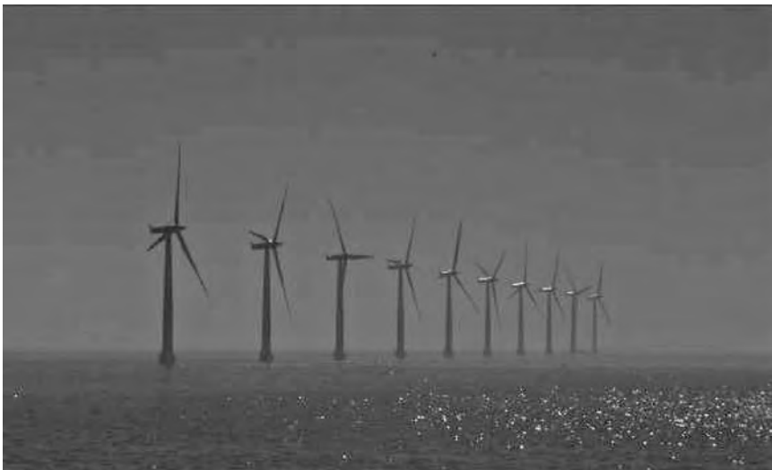
Plate 4.5.3 Offshore wind turbines ( Source: Samsø Energy Academy )
