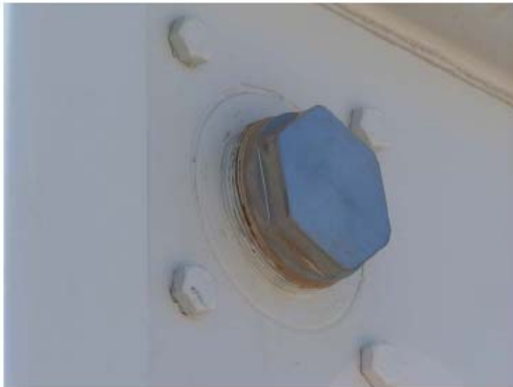
Figure 8: Tube end with flange threaded to tube neck and bolted to MEGC bulkhead
