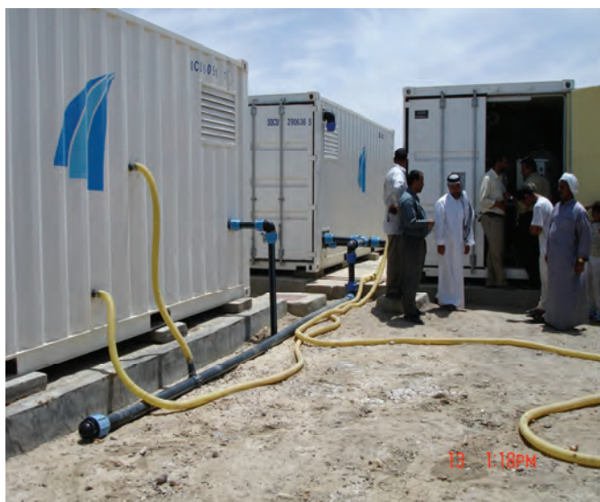
Figure 7 Water treatment facility during construction
