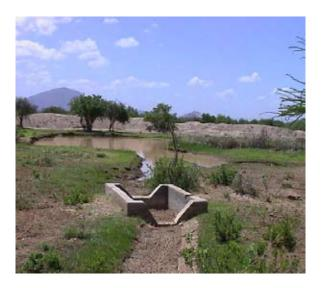
Photo (left): Silt trap intercepts sediments from the rainwater S Tumbo
