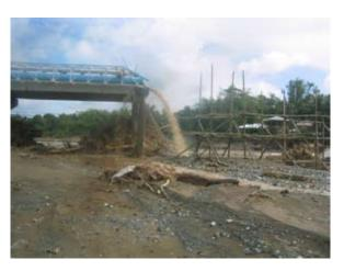
Flood-damaged main pipe for potable water for the City of Iloilo. Kahublagan
