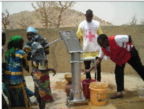
A water pump is restored in Zinder, Niger, as part of the Red Cross/Red Crescent WatSan project. Kinvi/International Federation
