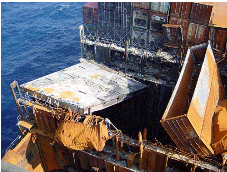
Image 4: MV Hanjin Pennsylvania – damage to hatch covers
