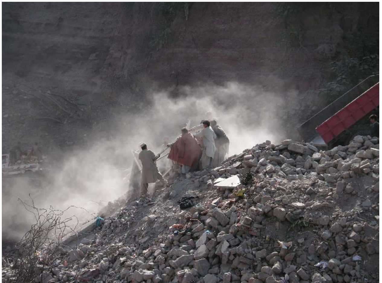
Debris being dumped in the earthquake aftermath (photo: L. Jönsson)
