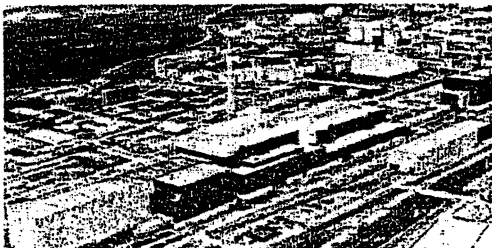
The Thermal Oxide Reprocessing Plant (THORP) at INEL. This commercial facility treats spent fuel from U.S. and overseas reactors, separating the high-level waste from uranium & plutonium. The smaller duct building on the right is the ventilation plant for the waste.
