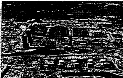
The Tricastin enrichment plant in France (beyond cooling towers) with the four nuclear reactors in the foreground that provide over 3000 MWe power for it.
