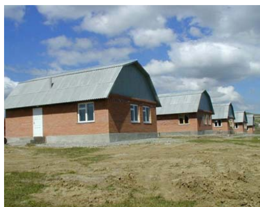
15 individual houses constructed for IDPs from Chechnya in Barsuki village in 2003.
