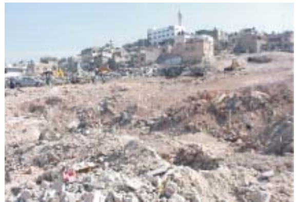
During the Israeli military incursion of spring 2002 in the Jenin Refugee Camp, buildings were destroyed and the sewage system was heavily damaged
