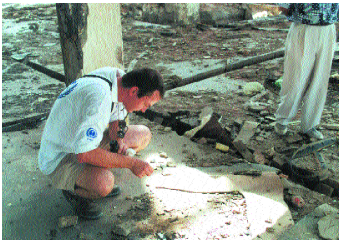
Site inspection at Vlorë complex
