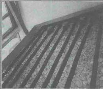
The upper filter bed, after installation but without plants
