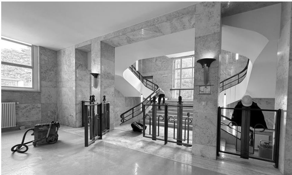
Figure III Application of protective varnish on handrails outside Hall XIV, building A
