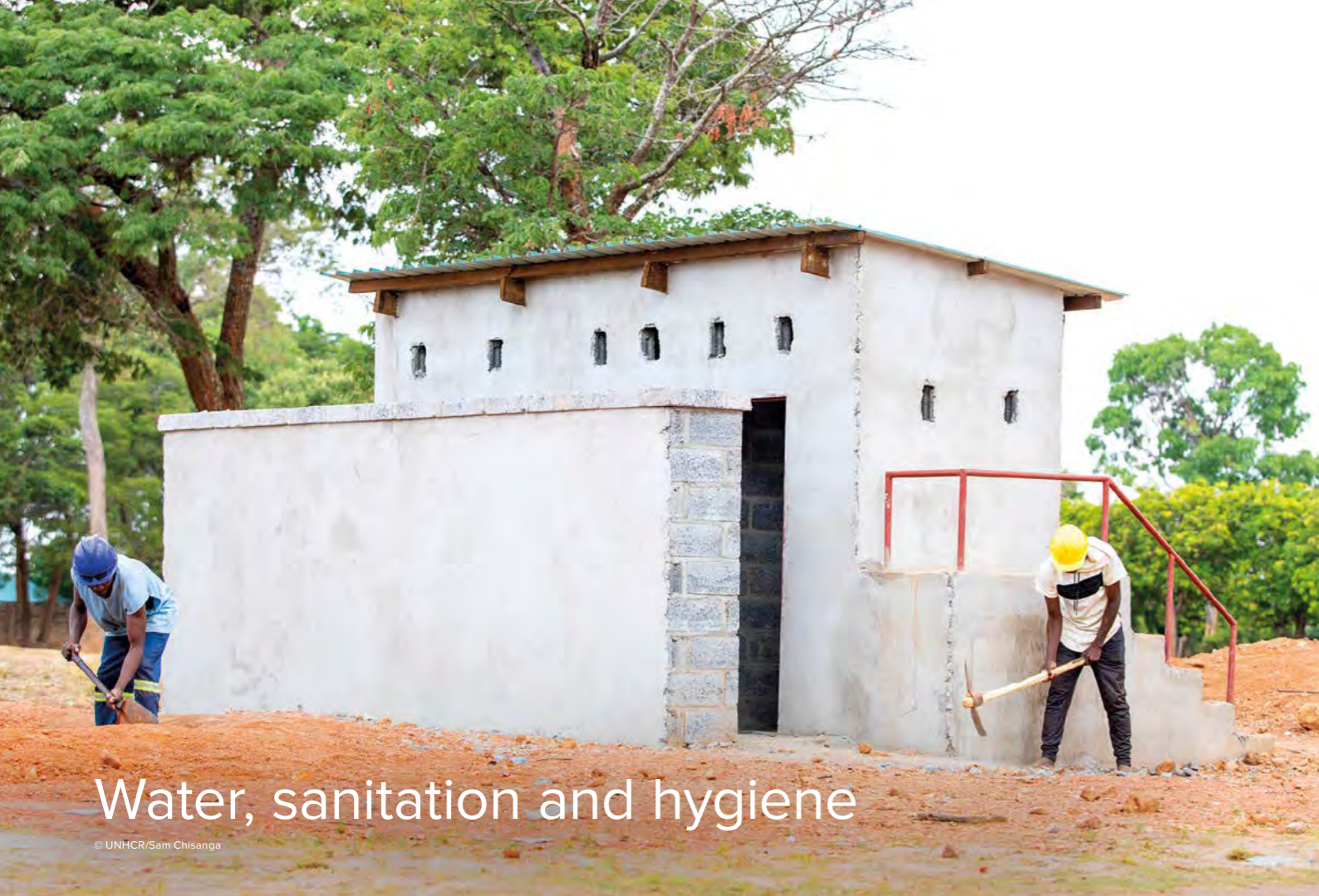
One of several ventilated improved pit latrines constructed in Meheba refugee settlement in Zambia, where they are being built to improve WASH facilities for people of concern.
