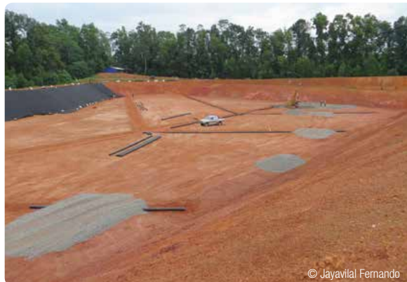
Sanitary landfill under construction
