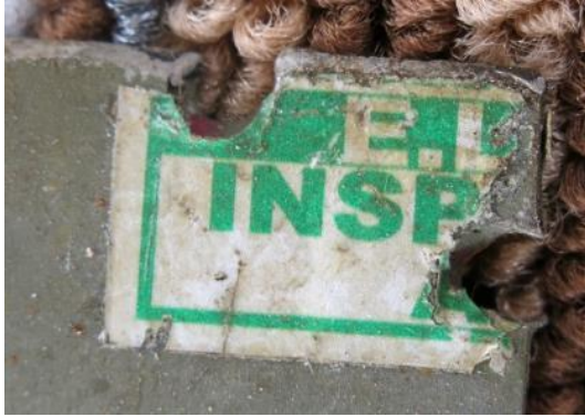
Figure 51.74. Close-up of a battery box part “E.L... / INSP.../A...” sticker
