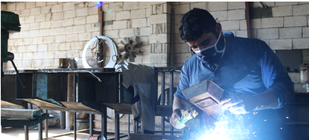
Maaret Al Ekwan Reception Center, Idlib. A man installs a boiler to provide heating for the winter months.
