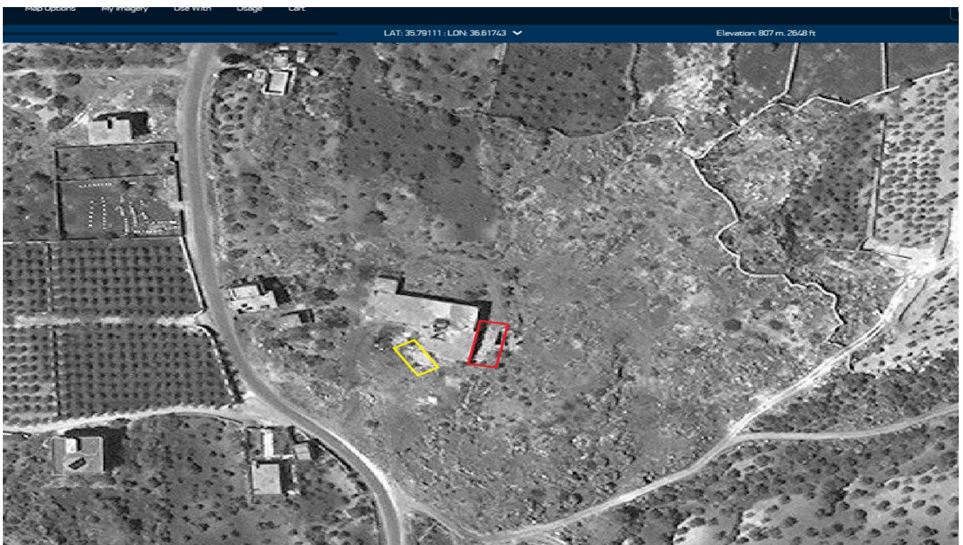
Satellite imagery showing damage to the building, 19 June 2022©2022 Maxar Technologies.
