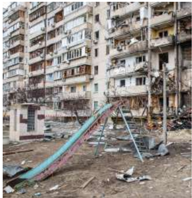
Damaged residential building, Kyiv, Ukraine © Drop of Light/Shutterstock
