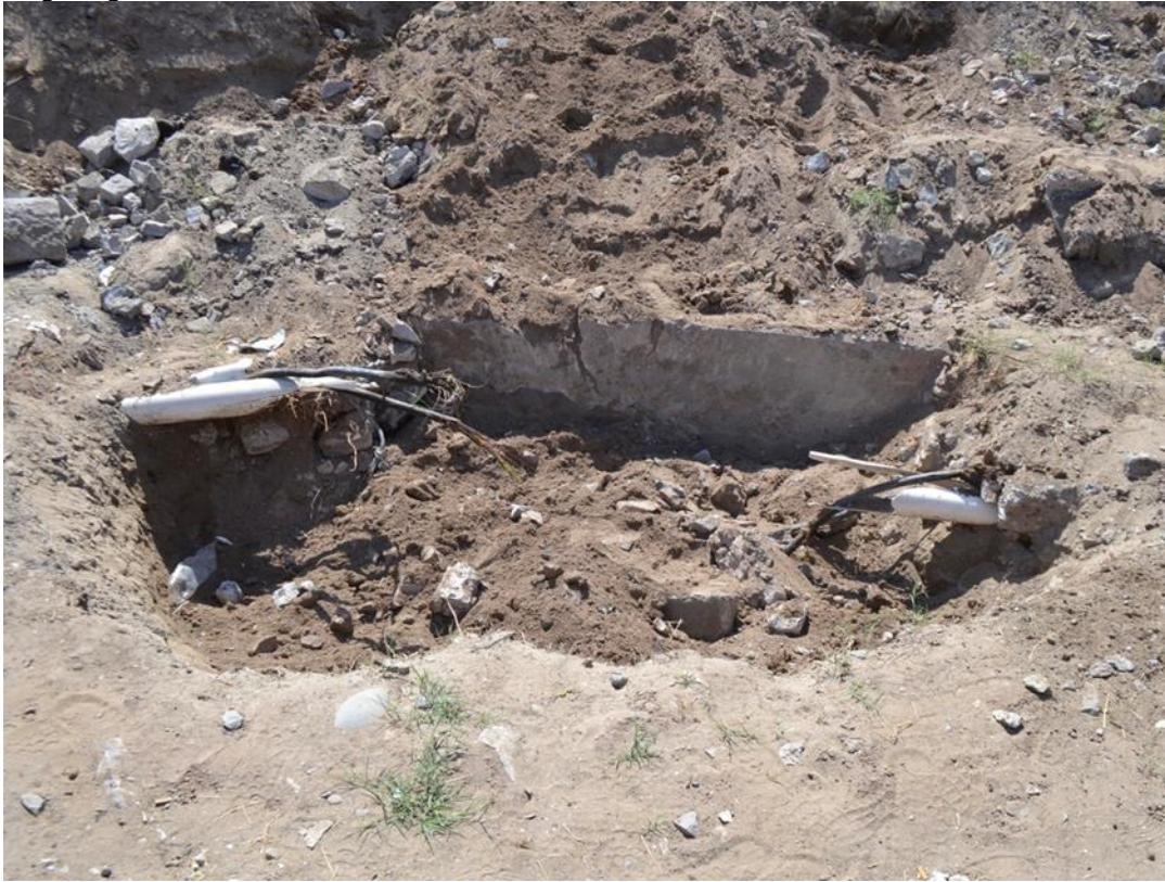
Figure 7.7 Impact point of the third missile on the low earth wall
