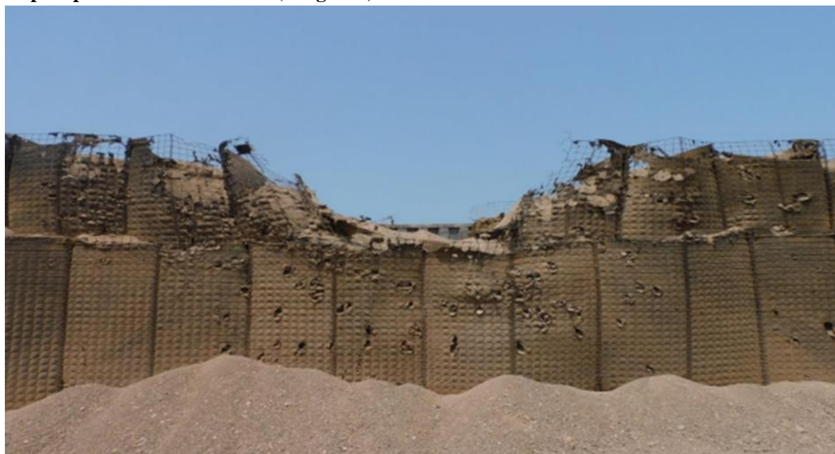
Figure 8.8 Impact point of the third UAV (Target #5)
