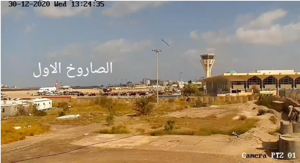
Figure 7.2 CCTV footage showing the impact of the first missile 30-12-2020 Wed 13:24:35
