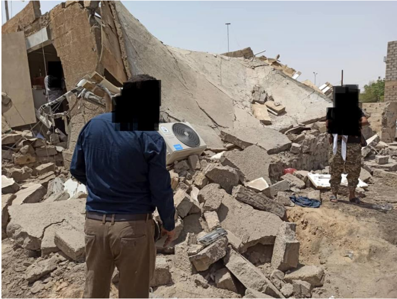
Figure 35.13 Damage to the Mosque
