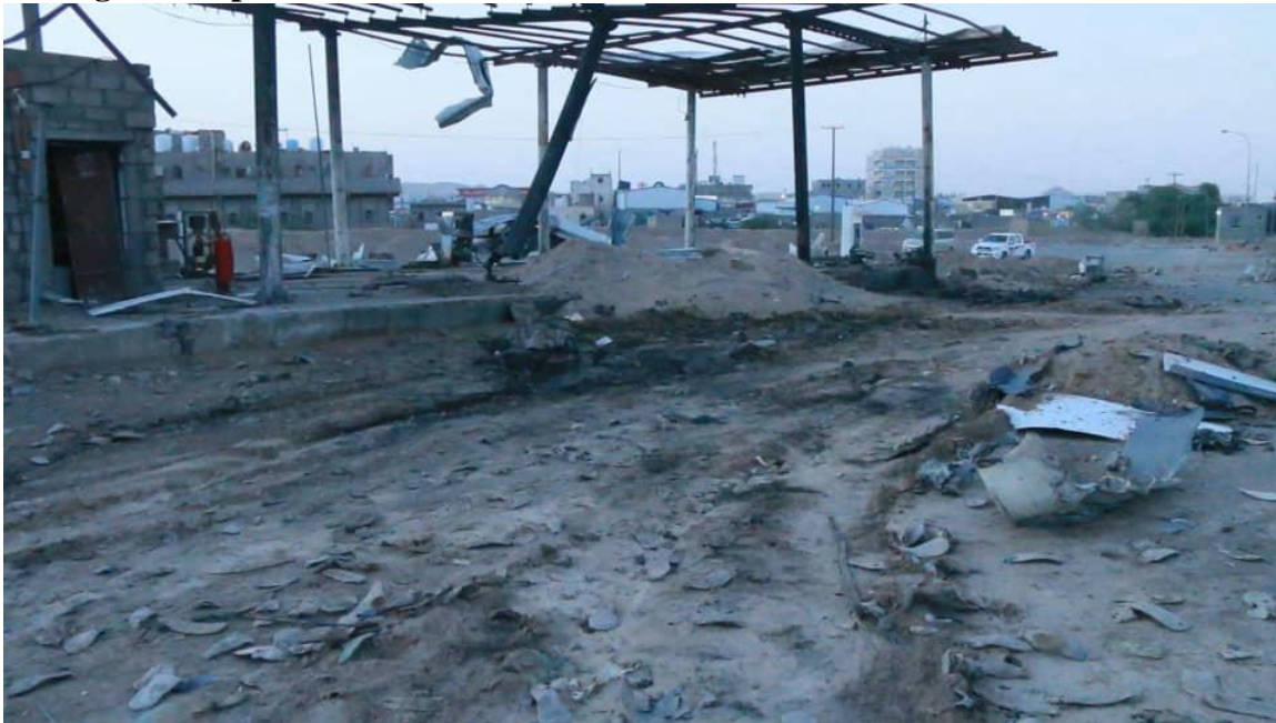
Figure 35.10 Damage to the petrol station
