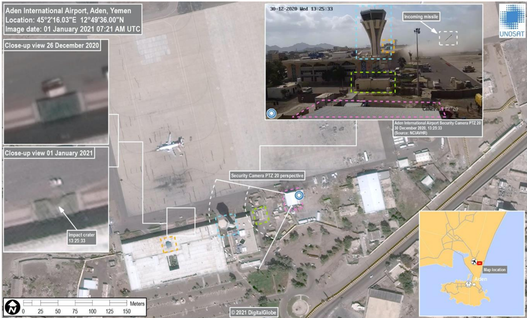
110/307 Figure 7.20 Satellite image of Aden Airport showing the location of the impact of the third missile
