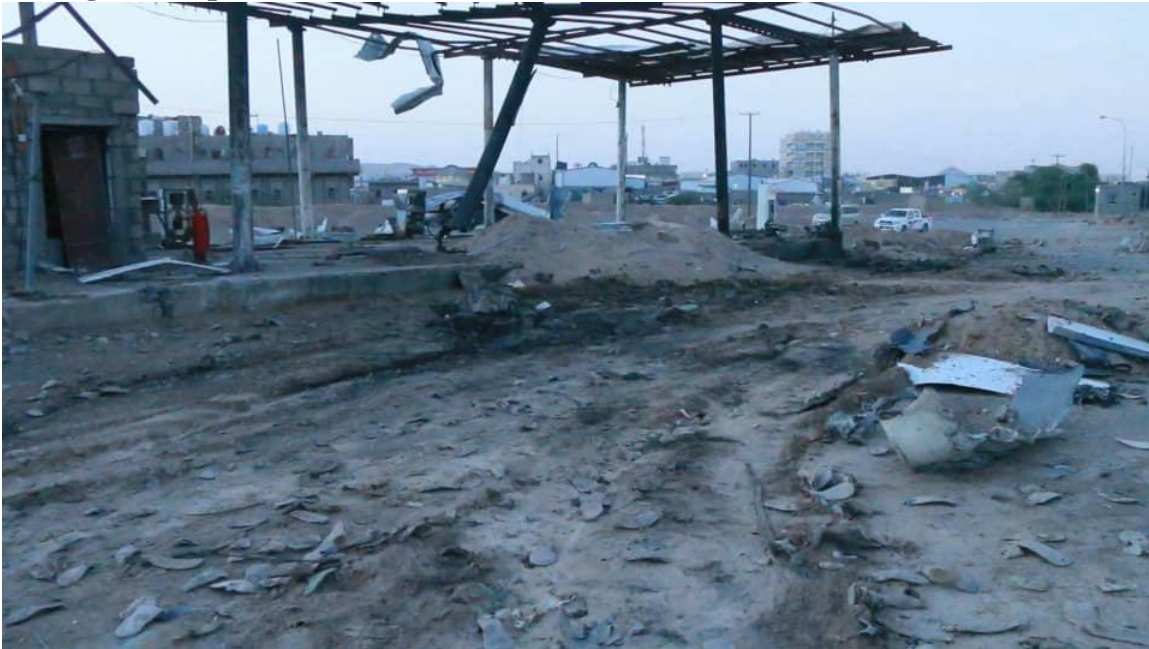
Figure 35.10 Damage to the petrol station
