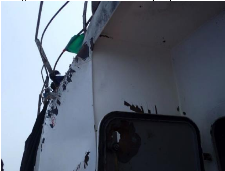
Figure 15.4 Damage to exterior bulkhead below the impact point
