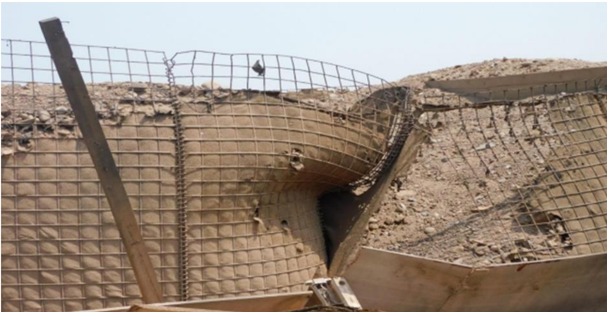
Figure 8.7 Impact point of another UAV and damage caused (Target #4)
