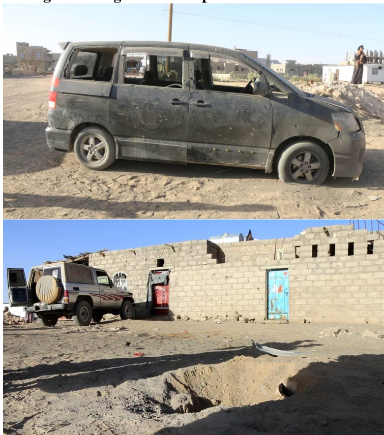
Figure 35.5 Damage resulting from the explosive ordnance
