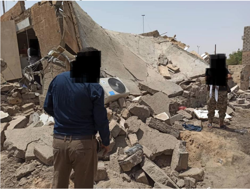
Figure 35.13 Damage to the Mosque
