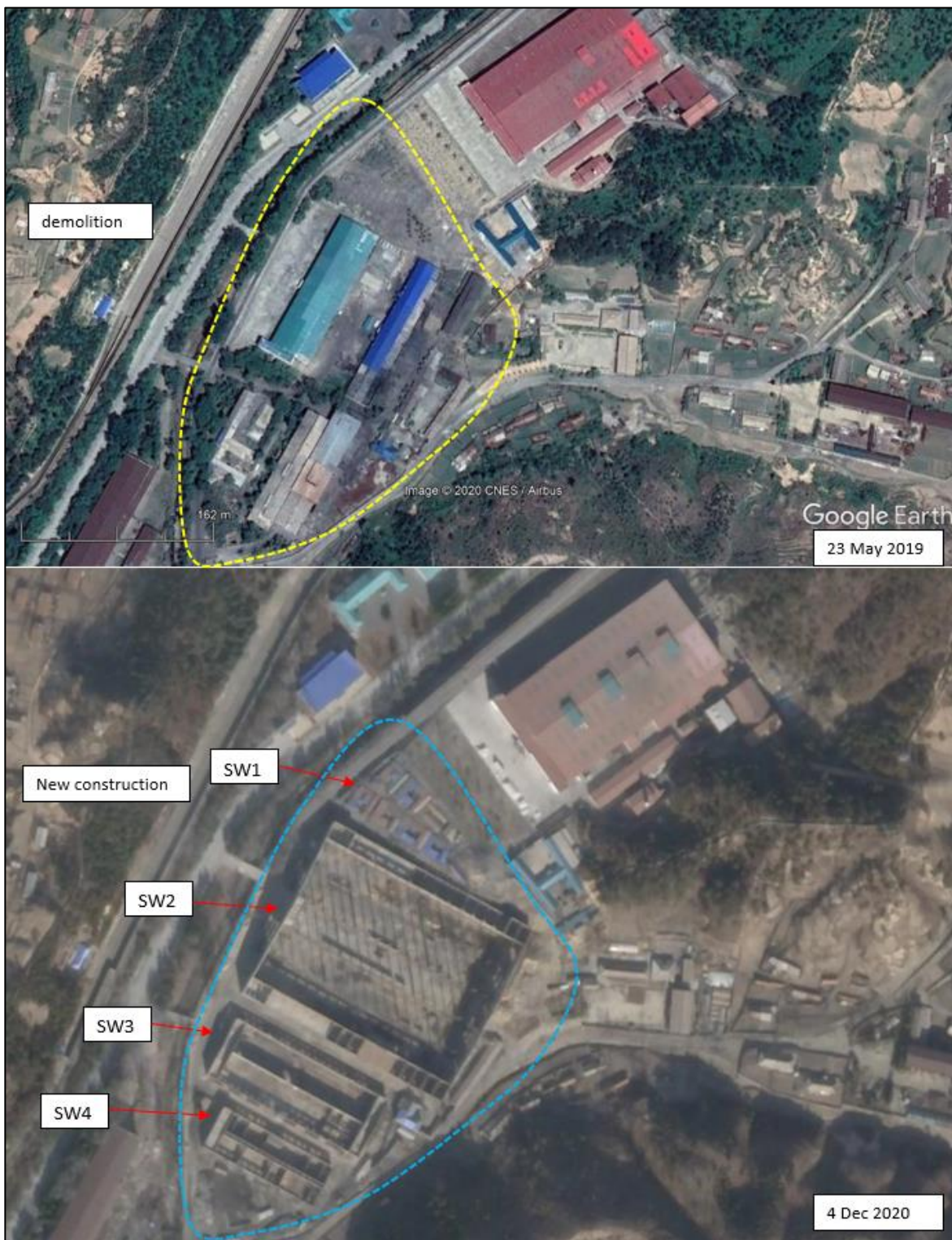
Figure 13-3: Focus on the demolition of several buildings and new constructions on the site SW (South-west corner: 40° 03' 17" N 125° 13' 16" E; Northeast corner: 40° 03' 26" N 125° 13' 29" EE) from Aug 2020
