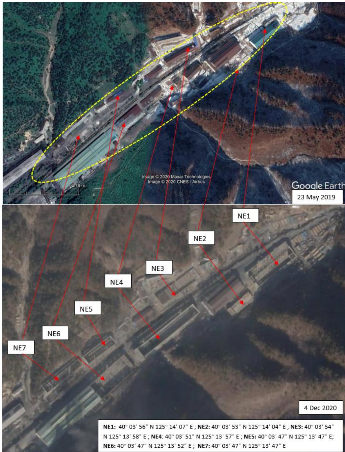
Figure 13-5: Focus on Demolition of several buildings and new construction on the site NE (southwest corner: 40° 03' 47" N 125° 13' 47"; northeast corner: 40° 03' 56" N 125° 14' 08" E) from Aug. 2020
