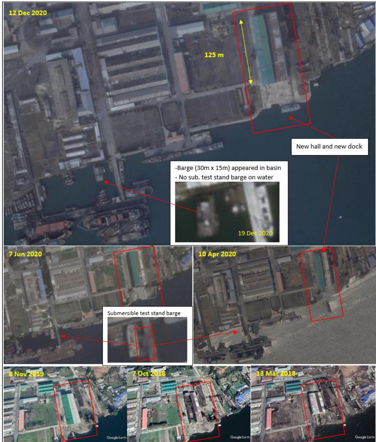
Figure 15-6: Nampo naval shipyard: renovation of the construction/maintenance hall (, 38° 43' 14" N 125° 23' 52" E) and activity inside secure boat basin (38° 43' 06" N 125° 23' 40" E)
