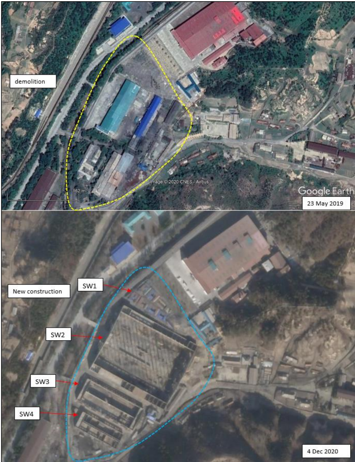
Figure 13-3: Focus on the demolition of several buildings and new constructions on the site SW (Southwest corner: 40° 03' 17" N 125° 13' 16" E; Northeast corner: 40° 03' 26" N 125° 13' 29" EE) from Aug 2020
