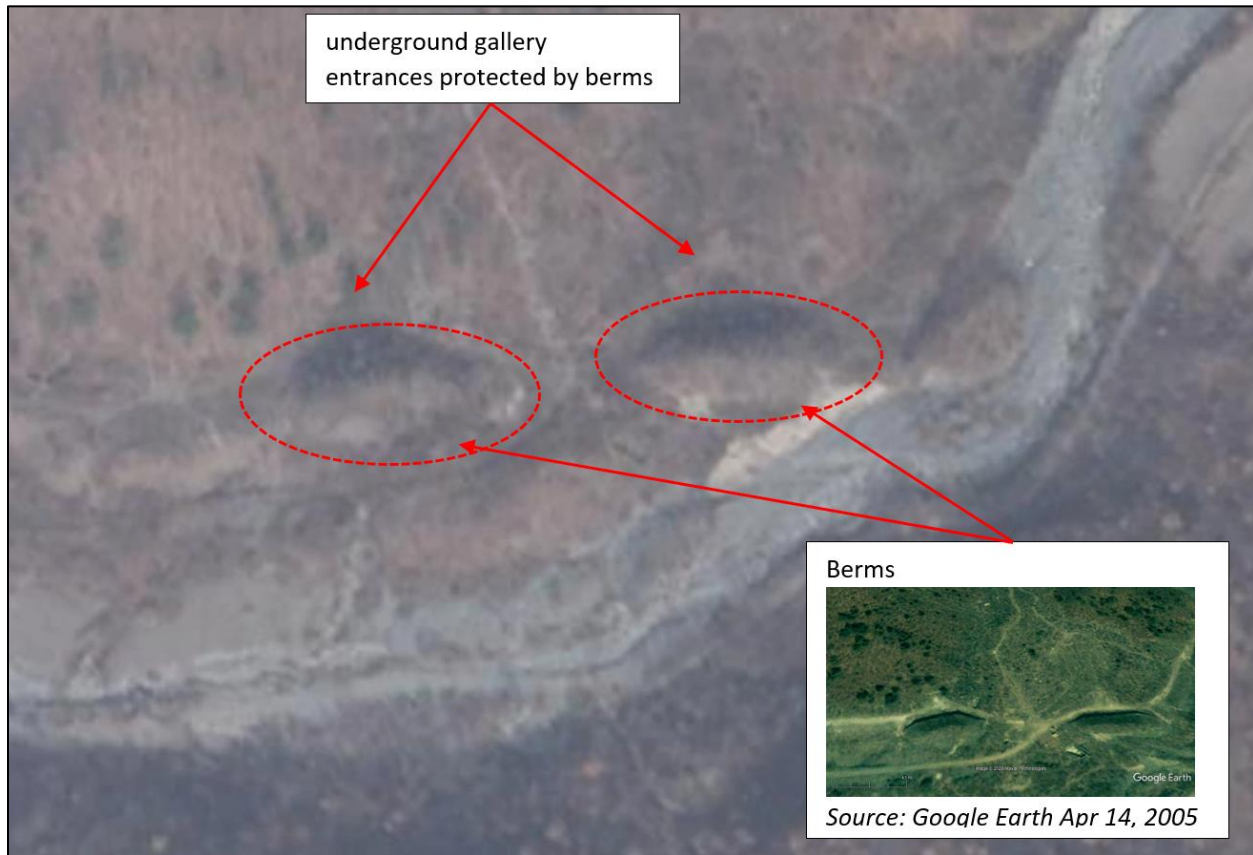
Figure 17-2: Kal-gol missile operating base two underground gallery entrances and their protective berms (location 38°40'10.93"N 126°45'23.57"E and 38°40'11.43"N 126°45'28.65"E).
