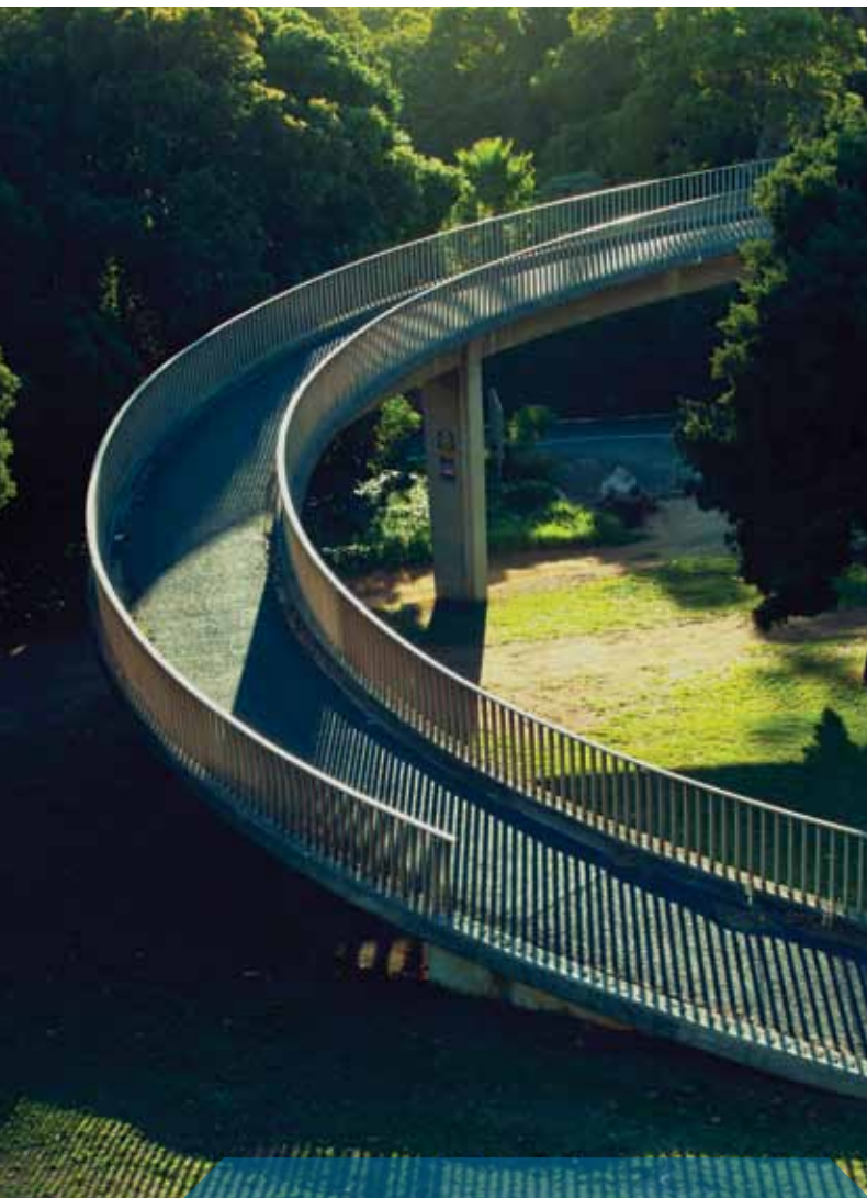
A pedestrian bridge (part of the railing stolen for scrap) near Cape Town, South Africa
