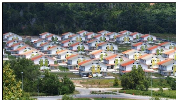
Image: One of the many residential areas under the National Housing Programme.
