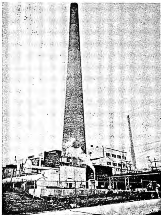
Figure 4. Stack and decontamination equipment for exhaust gases
