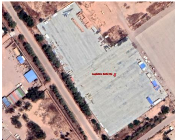
Figure 39.A.5 Misrata airport (13 May 2020)
