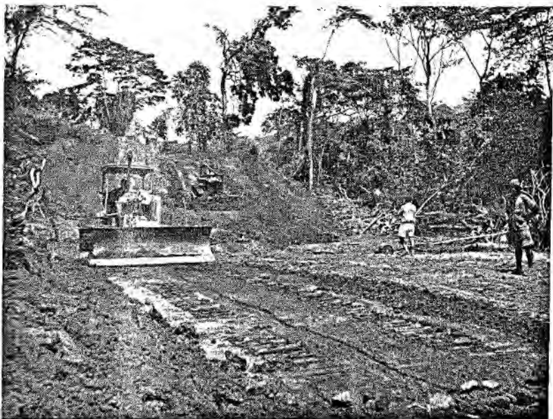
MPUNDU/TIKO RAILWAY UNDER CONSTRUCTION
