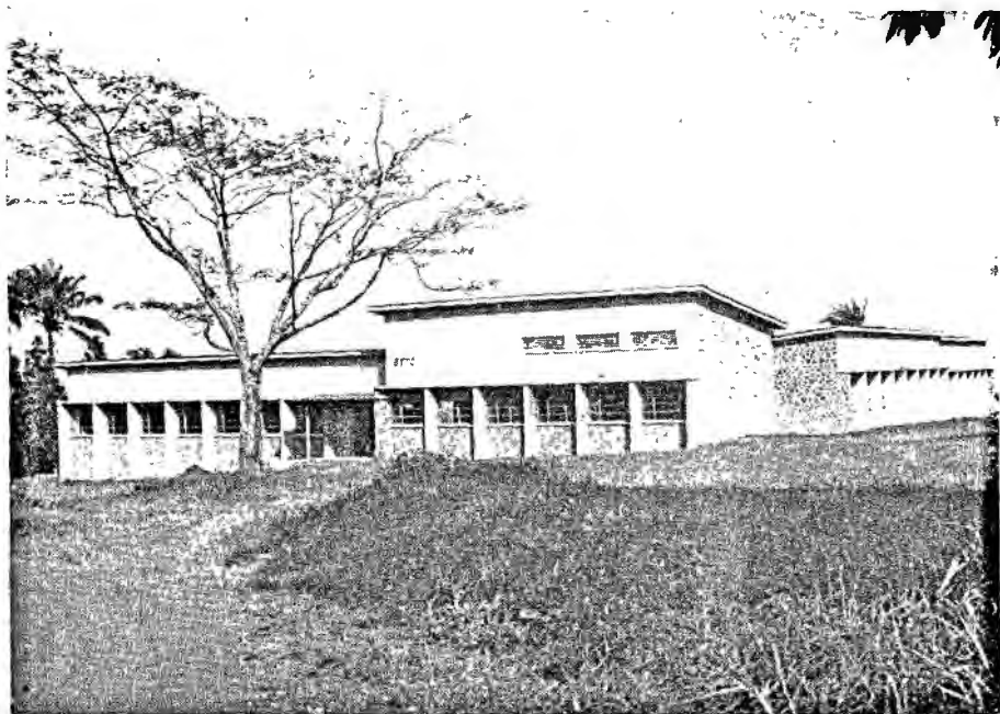
A newly constructed building of the Baptist Teacher Training Centre at Great Soppo, Buea.
