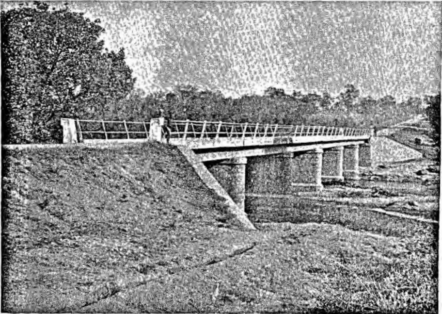
New bridge construction, Berli-Serti Road, 1957.
