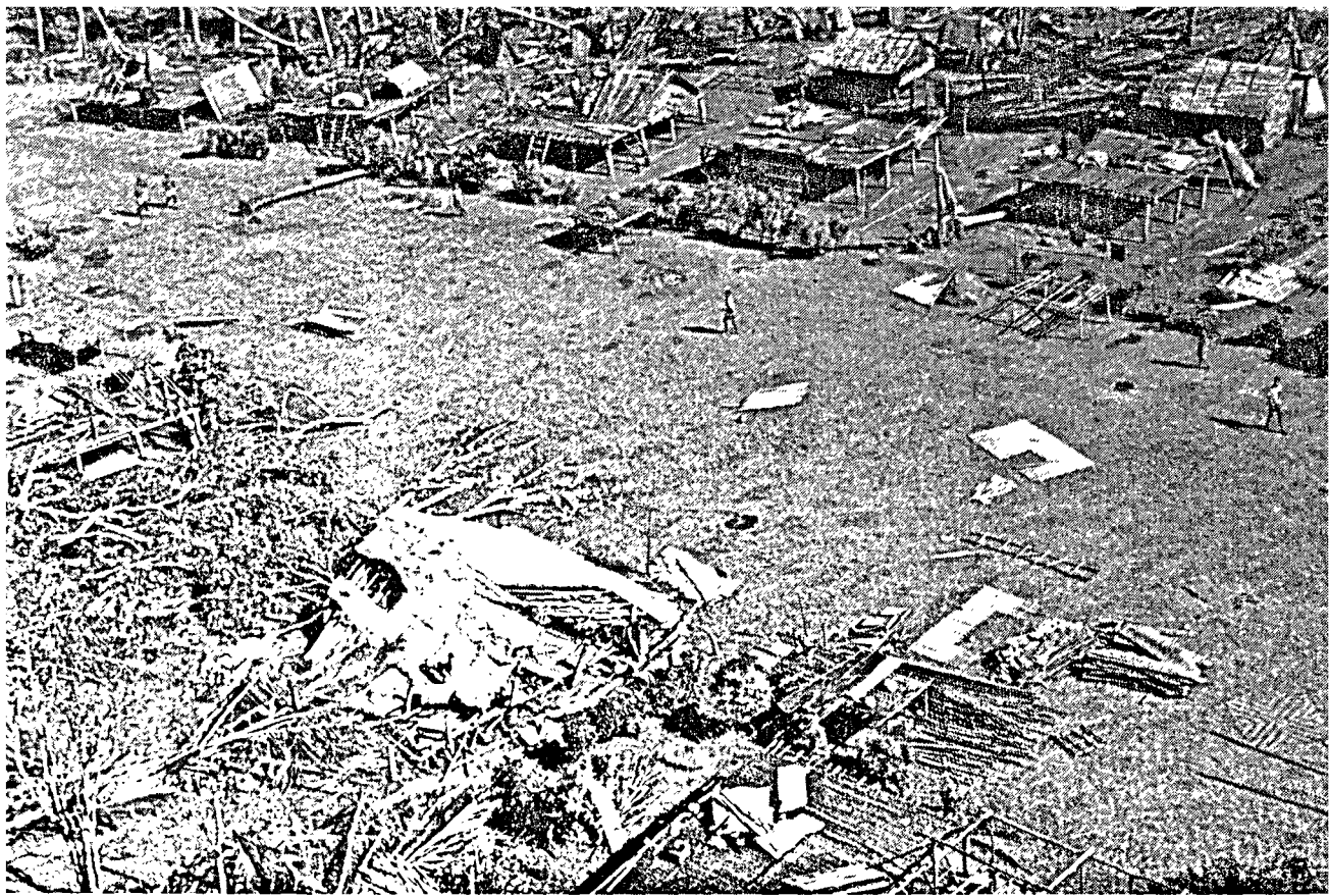
(Above) Cyclone damage at Tufi in the Northern District.
