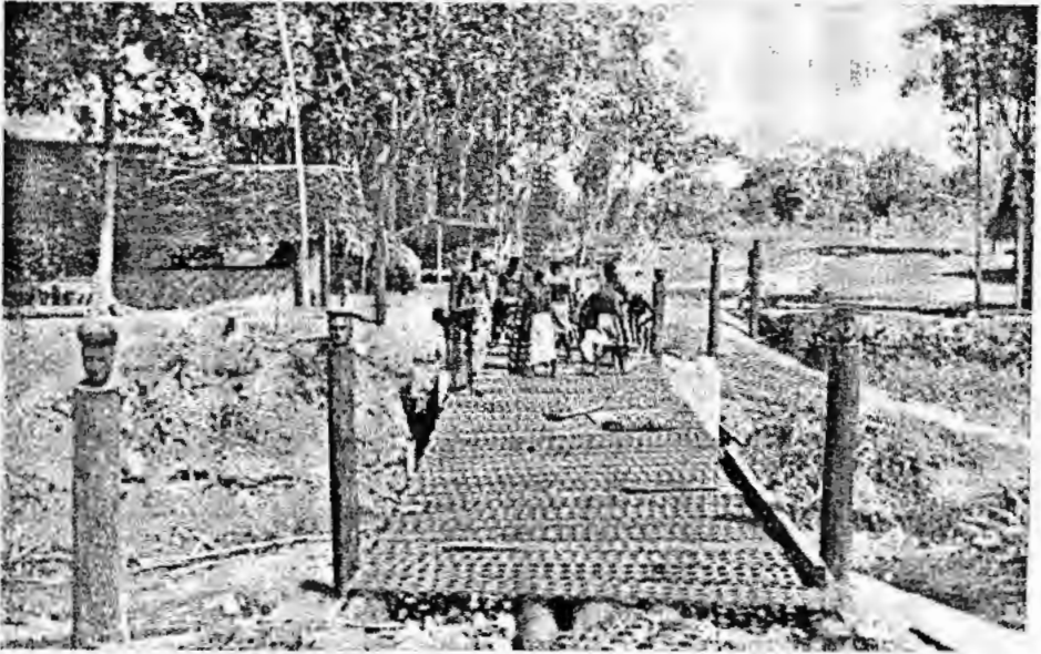
Bridge under construction—Gogol Valley road.
