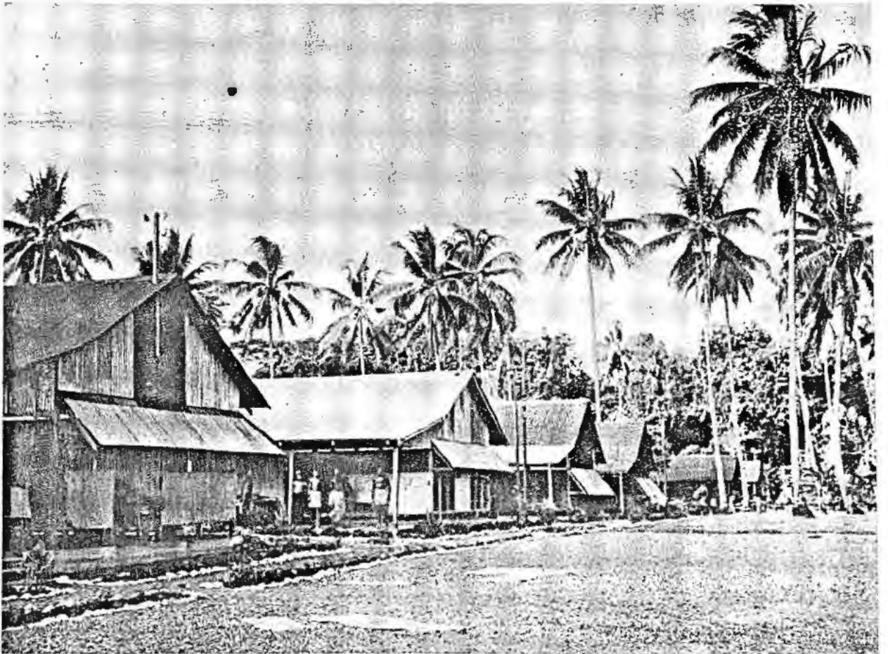
Native hospital at Lae.
