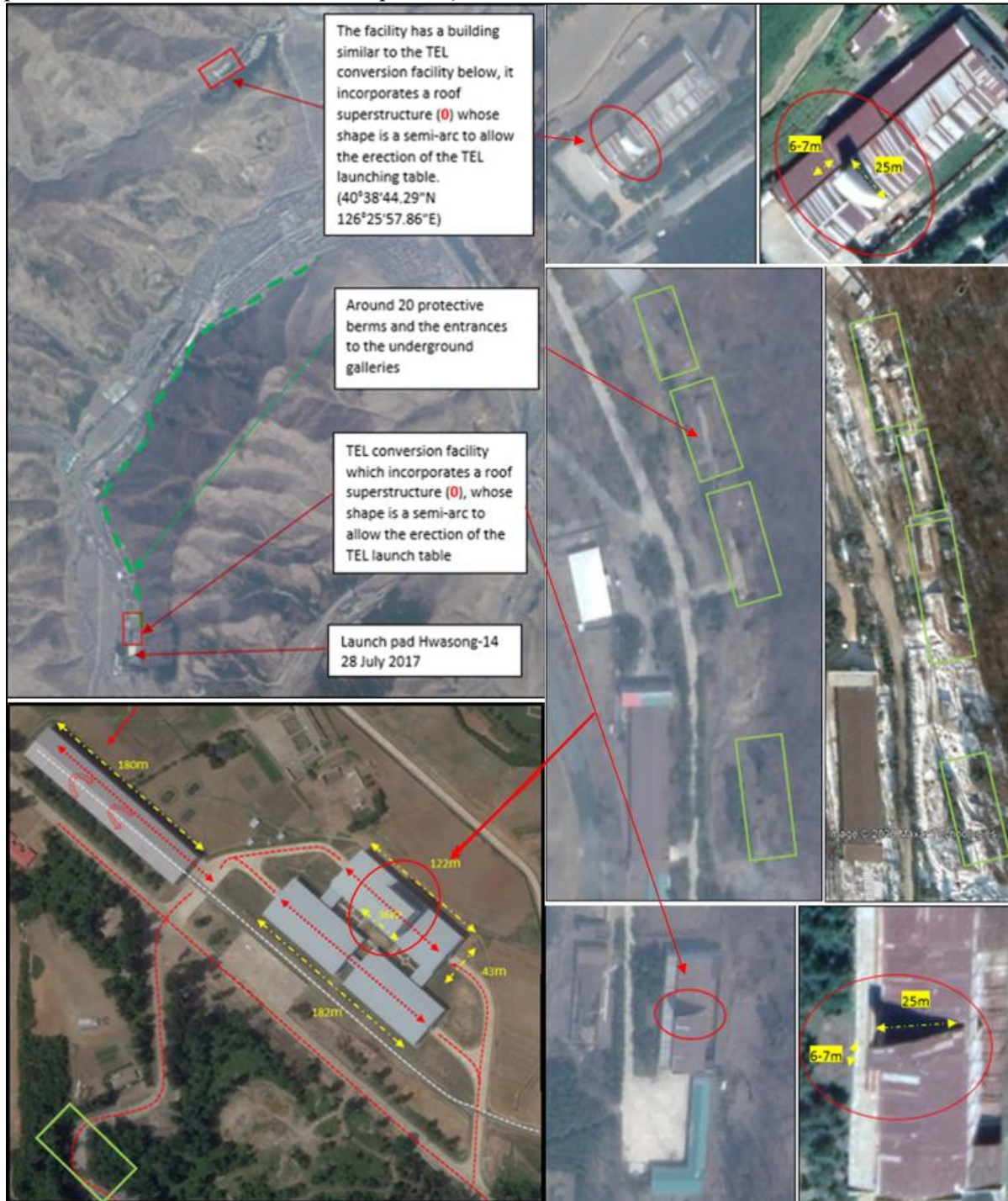
Figure 12-9: Comparison between structure of the possible ballistic missile support facility (aka Sil-li ballistic missile support facility) (39°10'50.56"N 125°39'50.01"E) and at the Jonchon-Mupyong-ni No 65 factory , the southern building involved in the TEL upgrading (40°36'42.77"N 126°25'34.74"E) and the various underground galleries located along the westside of the mountain from south (40°36'48.06"N 126°25'35.59"E) to north-east (40°38'0.43"N 126°26'21.20"E). A Hwasong-14 was tested on 28 July 2017 from a near-by launch pad (40°36'40.21"N 126°25'33.31"E) (see S/2019/171, para. 174; S/2018/171, paras. 9,11,12 and 13; S/2017/742, para. 7)
