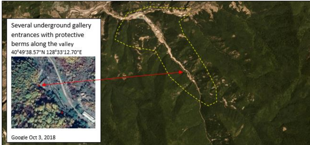
Figure 9-6: Sangnam-ri Missile operating base activity (40°50'7.46"N 128°32'47.42"E). Con-firmed underground gallery entrances are located along the valley from - 40°49'35.89"N 128°33'15.41"E - 40°49'38.57"N 128°33'12.70"E - 40°49'42.22"N 128°33'9.32"E - 40°49'43.90"N 128°33'7.39"E – are identifiable because of the protective berms in front.
