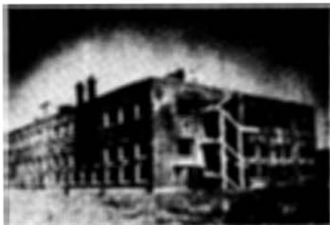
No. 11. The lateral and front view of the main production building where most of the new equipment were installed.
