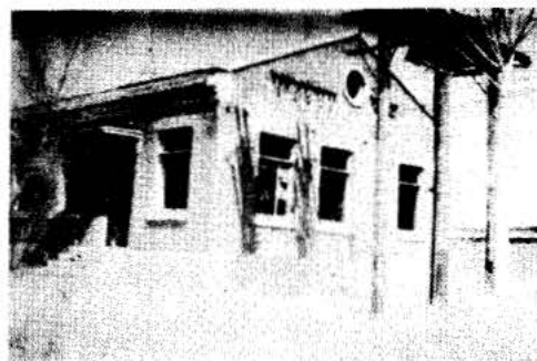
No. 6. This is the house for the power units.
