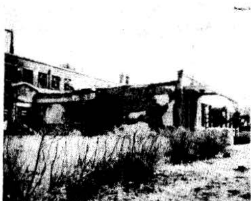
No. 5. Another half of the building that the bombs missed.
