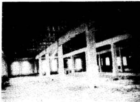
No. 27. Shows the interior of a just completed factory, where installations have not been assembled. The roof of this building is in good condition.
