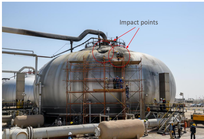
Figure 14.1 Damaged separator tank in Abqaiq
