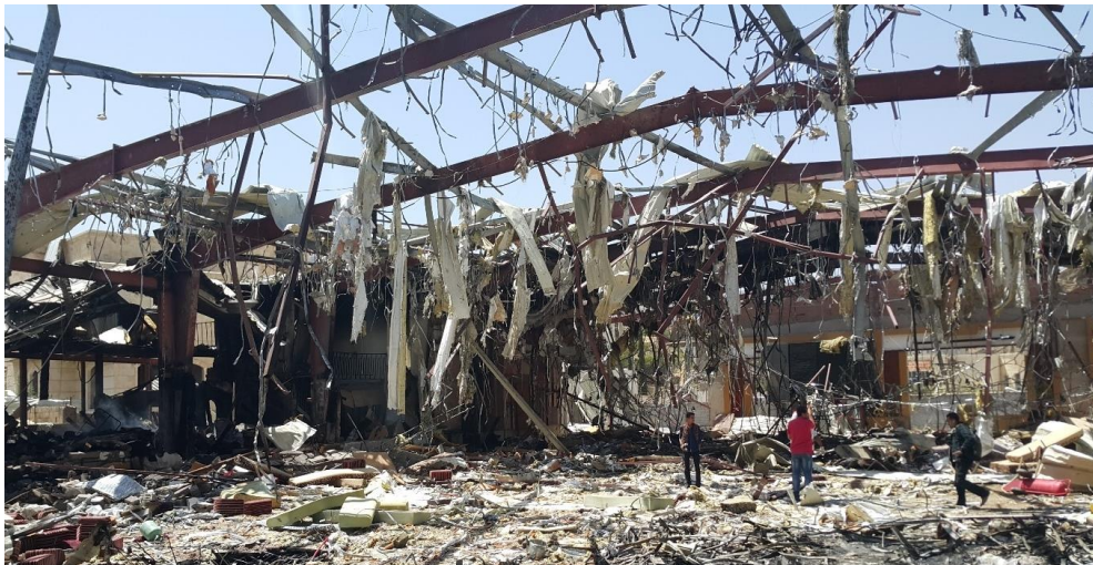
Destruction caused to Al Kubra Hall on 8 October 2016 2
