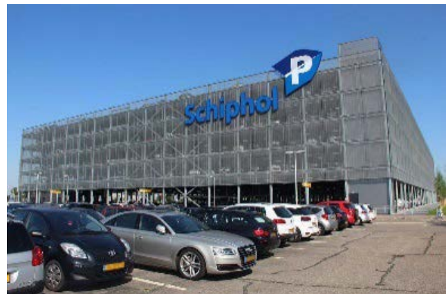
FIGURE 4: Demountable car park at Schiphol Airport
