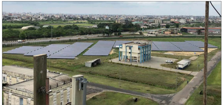
FIGURE 1: Solar-at-Gate project installation at Douala International Airport, Cameroon
