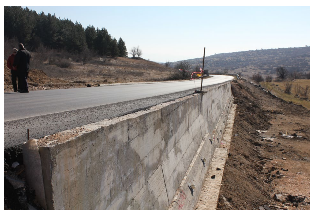
Photo 7c: Repairing the road after a landslide
