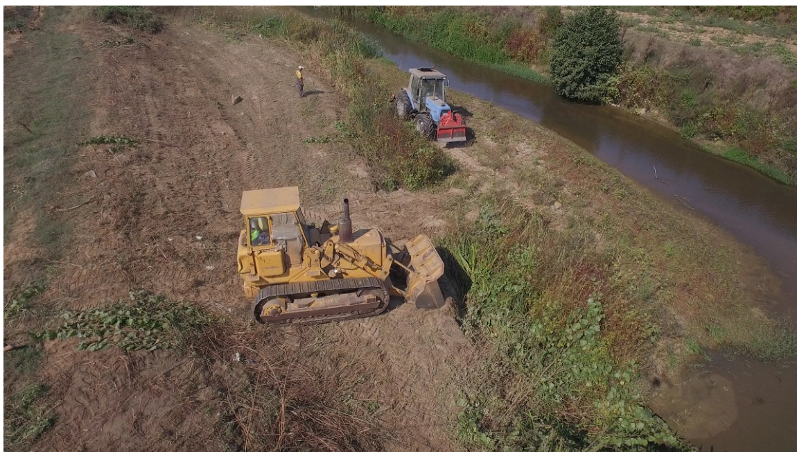
Photo 2b: Cleaning the riverbed
