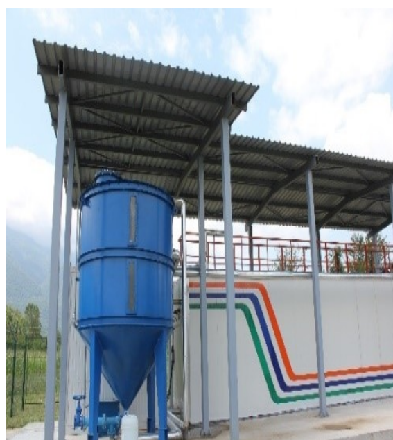
Photo 9b: Wastewater treatment plant in Novo Selo
