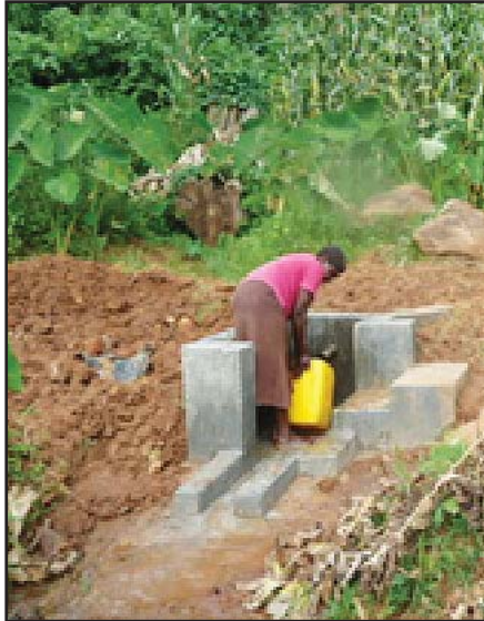
Woman using new water spout after the construction of spring protection
