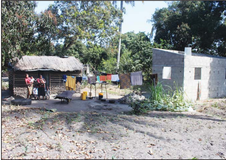
Old house and new house under construction
