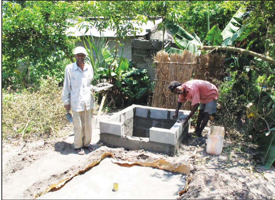
Building an approved latrine
